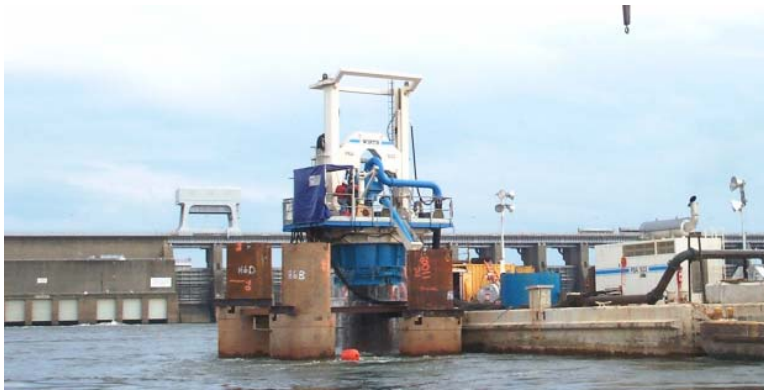
Figure A-120. Wirth pile top reverse circulation drill.
