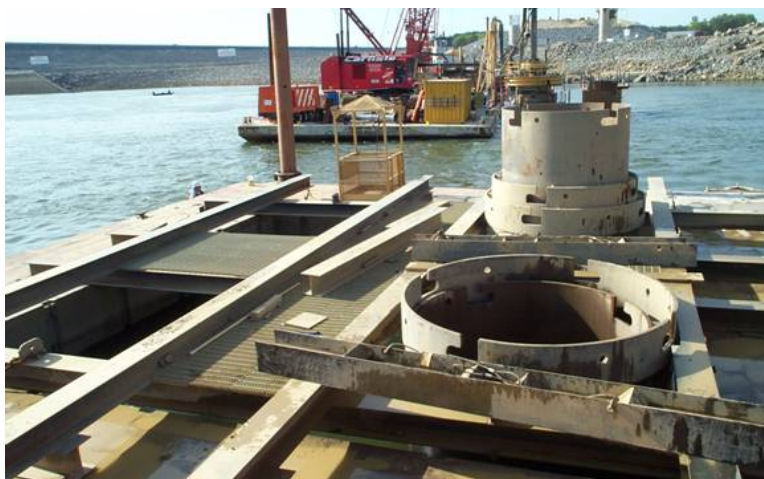
Figure A-122. Permanent casing set inside temporary casing.
