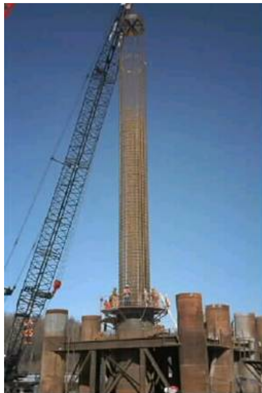
Figure A-69. Typical reinforcement installation using lifting ring and crane.
