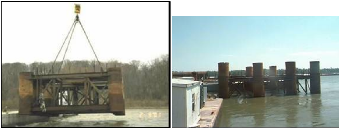
Figure A-63. Nose pier template.
