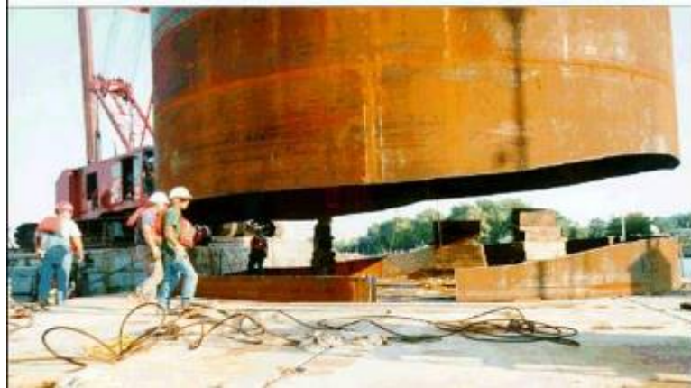
Figure A-108. Bottom of cell scribed and cut to match rock surface.
