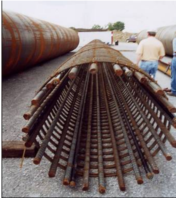
Figure A-127. Rebar cage with CSL tubes. Figure A-128. Placing tremie concrete.
