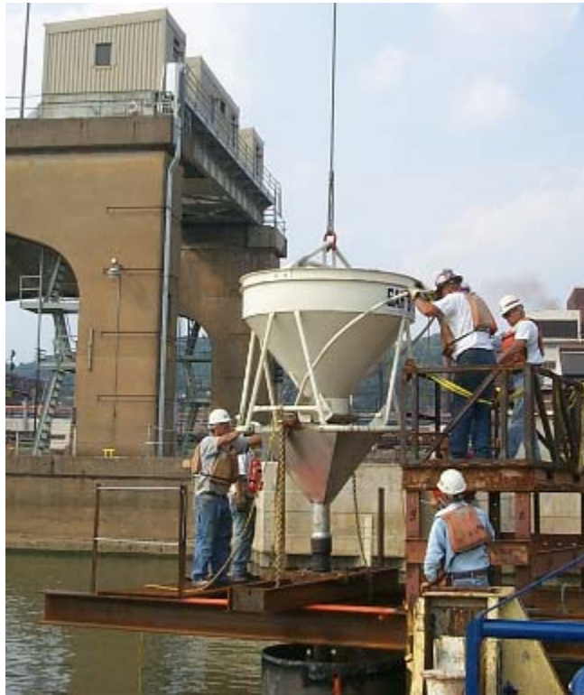
Figure A-93. Drilled shaft concrete placement by tremie method.
