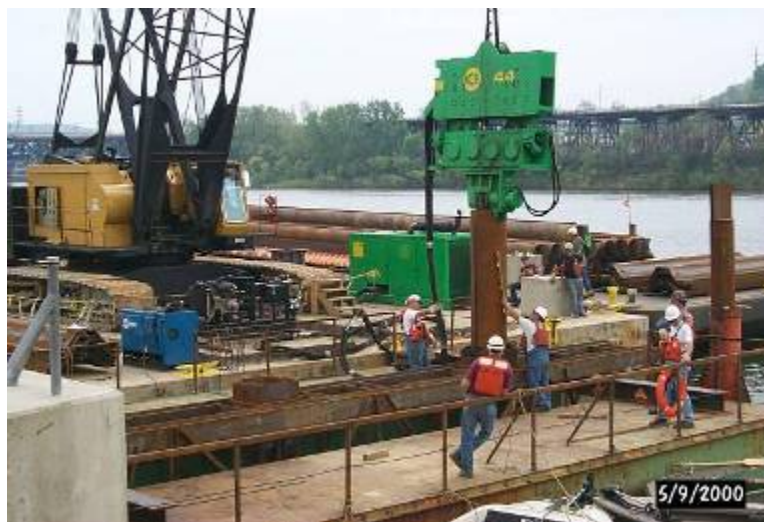
Figure A-83. Driving downstream cut-off wall master piles.
