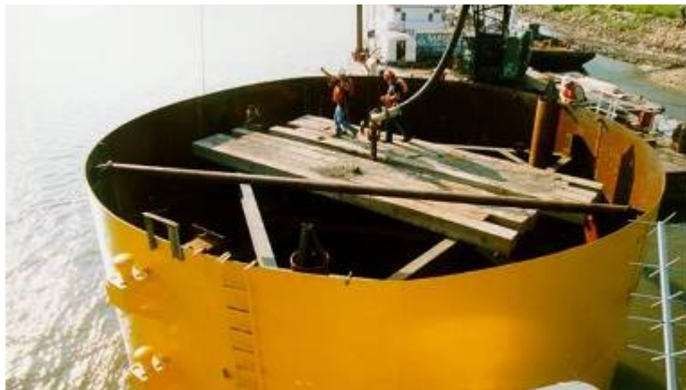
Figure A-112. Placing tremie concrete.
