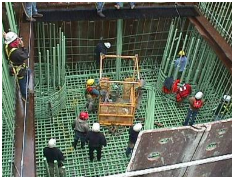
Figure A-16. Bath-Woolwich Bridge dewatered cofferdam.
