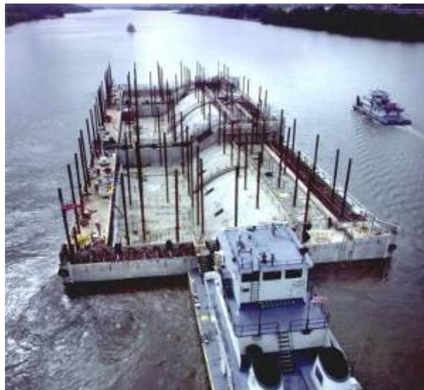
Figure A-6. First dam segment under tow up the Monongahela River to Braddock Dam.
