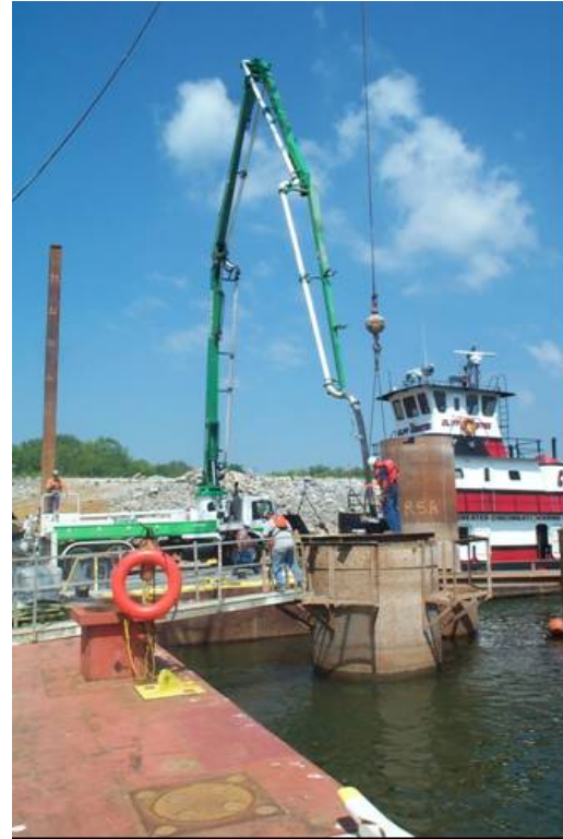
Figure A-127. Rebar cage with CSL tubes. Figure A-128. Placing tremie concrete.
