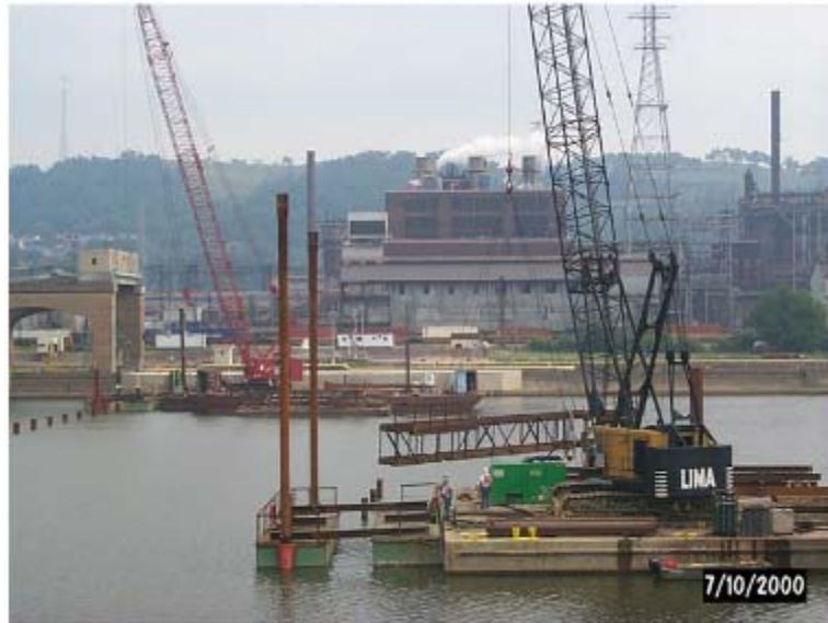
Figure A-79. Assembly of floating guide frame.
