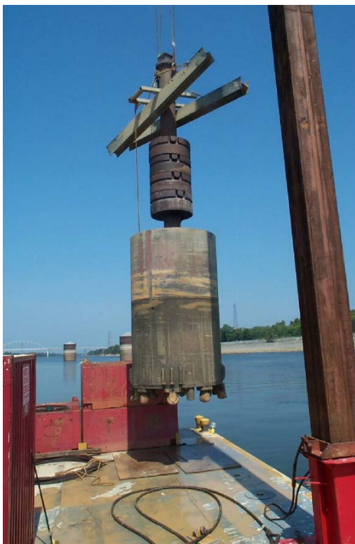
Figure A-118. Kerf cutting bit.
