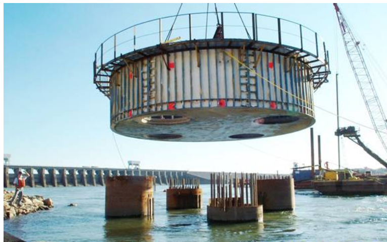
Figure A-129. Setting pier base form.
