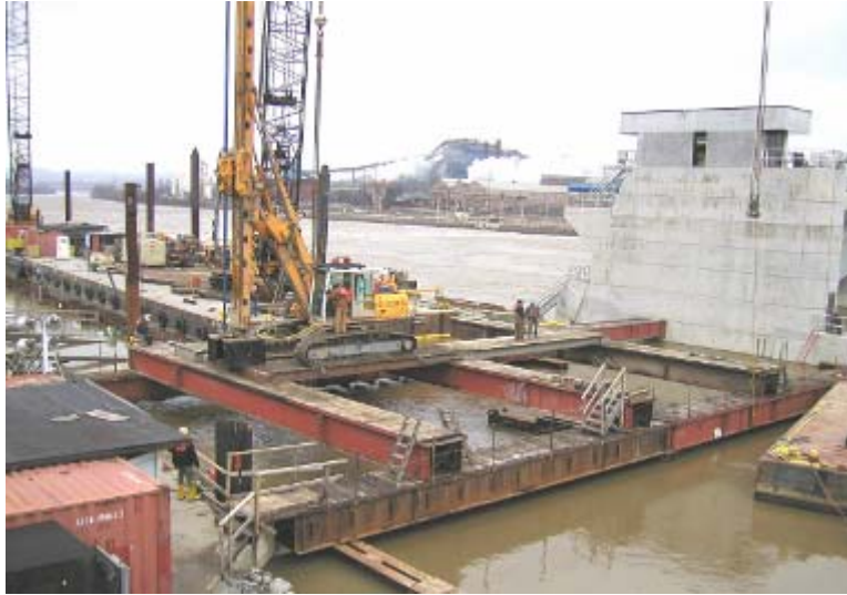
Figure A-103. Rotary drill rig with monitor with temporary work trestle.
