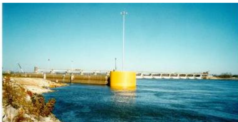
Figure A-113. Downstream view of completed cell.
