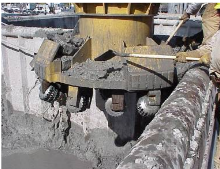
Figure A-46. Rotary cone drill bits used on the New Carquinez Bridge.
