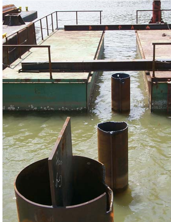
Figure A-28. King-piles floating template.
