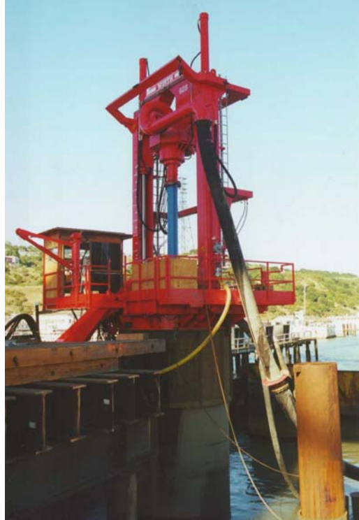
Figure A-44. Pile-top drill rig used for 10-foot-diameter drilled shafts on the New Carquinez Bridge.
