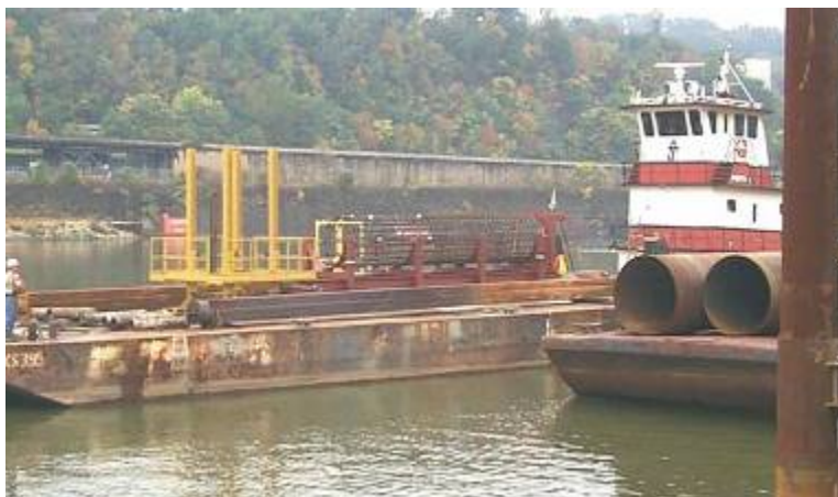
Figure A-91. Drilled shaft reinforcing cage ready for installation.
