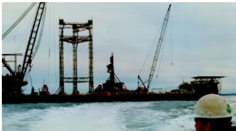
Figure A-18. Guide towers used to establish landing points for precast bridge piers on rock at Confederation Bridge.
