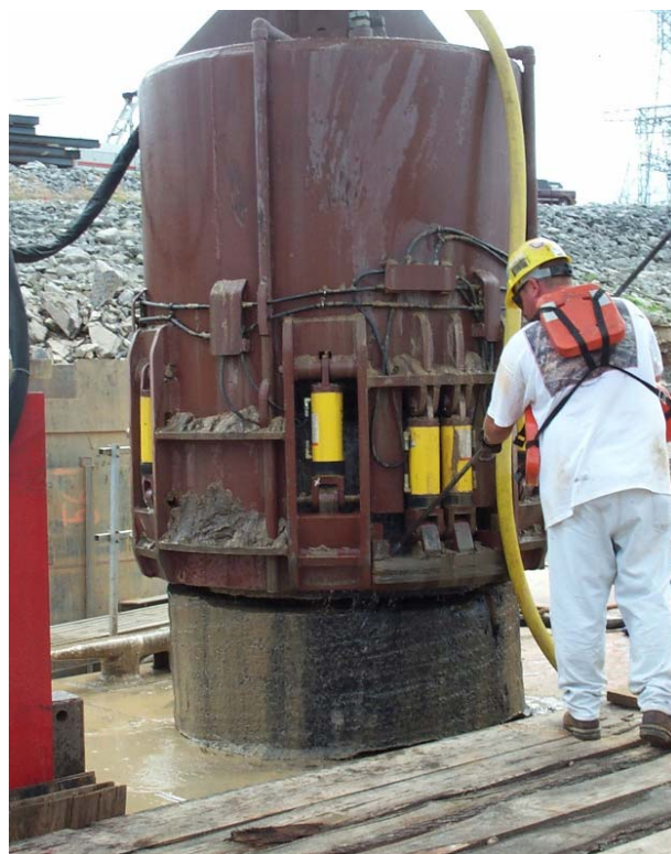
Figure A-119. Kerf core retriever.
