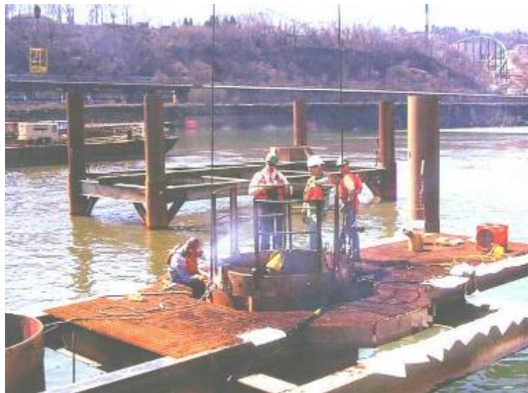
Figure A-97. Installation of coffer pipe for casing cut-off.
