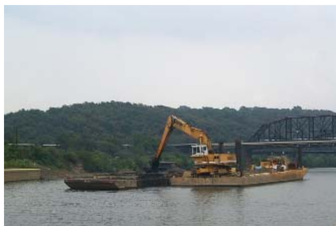
Figure A-75. Pre-excavation at dam's footprint.
