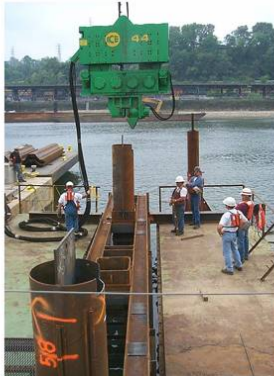
Figure A-82. Driving downstream cut-off wall master piles using floating guide template.
