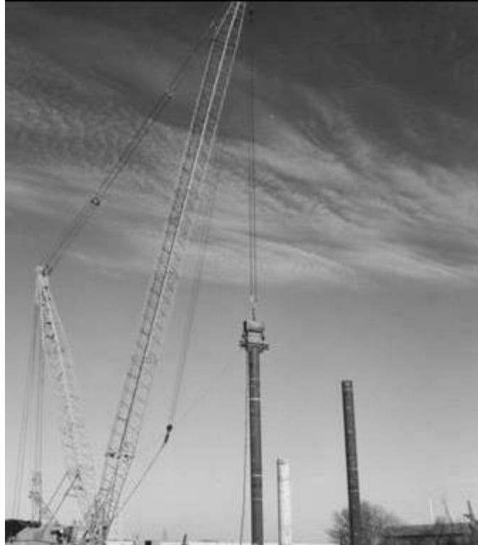
Figure A-72. Pile-mounted submersible hammer.
