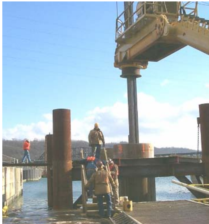
Figure A-90. Clean out of drilled shaft casing.
