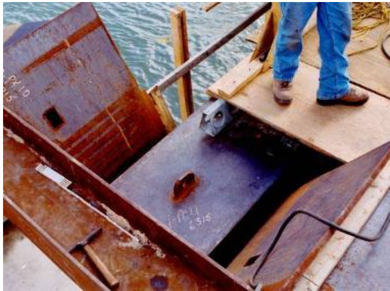
Figure A-15. Bath-Woolwich Bridge cofferdam being dewatered.
