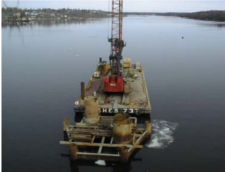
Figure A-17. Pile template and temporary casings used on the Bath-Woolwich Bridge.
