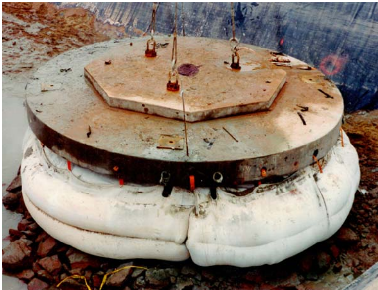
Figure A-20. Inflated grout bags at test landing point, Confederation Bridge.
