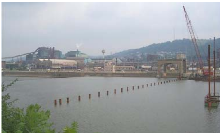
Figure A-84. Downstream cut-off wall master piles—24-inch-diameter pipe.
