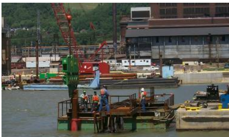
Figure A-27. Installing king-piles for underwater cutoff wall at Braddock Dam.
