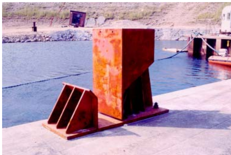
Figure A-4. Detail of horn-guide used on the Oresund Immersed Tube Tunnel.
