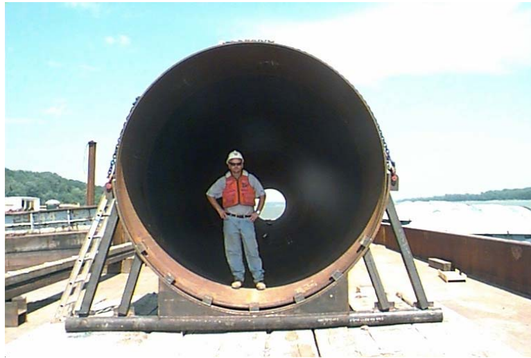
Figure A-62. Shaft casings with 10-foot diameter.
