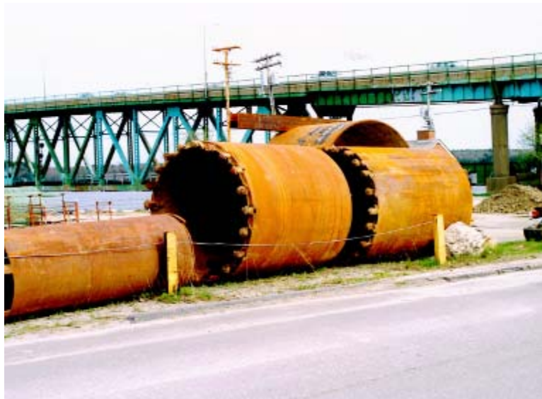
Figure A-42. Double wall shot barrel drill tools at Bath-Woolwich Bridge.
