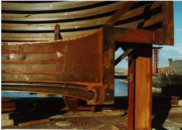
Figure A-35. Local section of pile top cofferdam for underwater cutoff of piles or casings.
