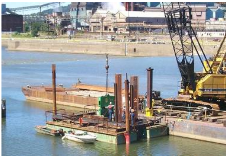
Figure A-85. Driving sheets for left side cut-off wall.
