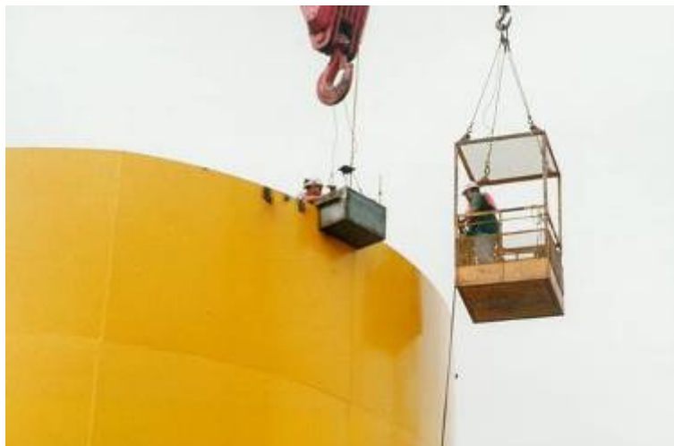
Figure A-107. GPS sensor on steel cell.
