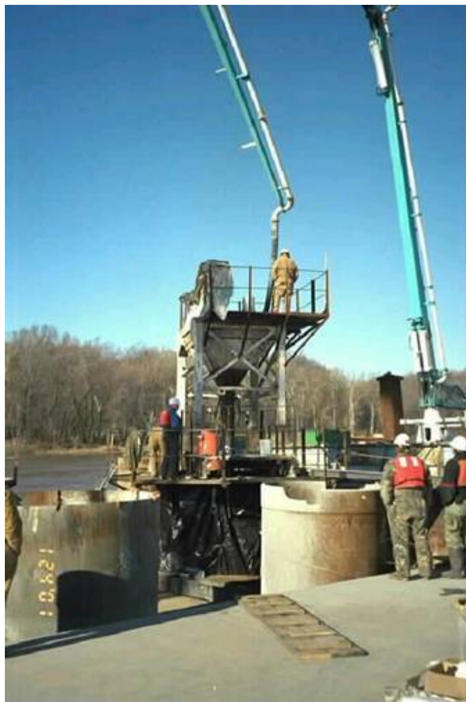
Figure A-70. Tremie concrete placement.
