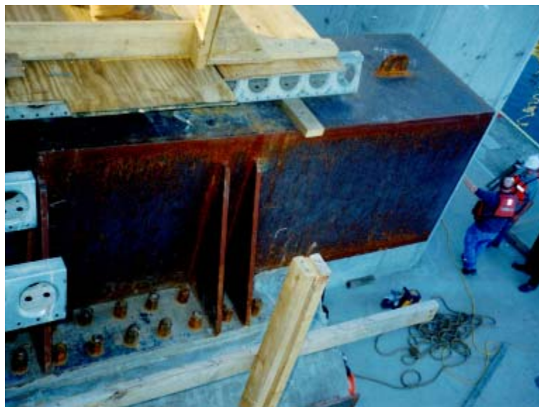
Figure A-37. Side view of male guide arm positioned above the horn-guide at Braddock Dam.
