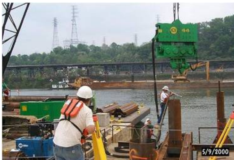
Figure A-80. Using master piles to monitor alignment of cut-off wall.
