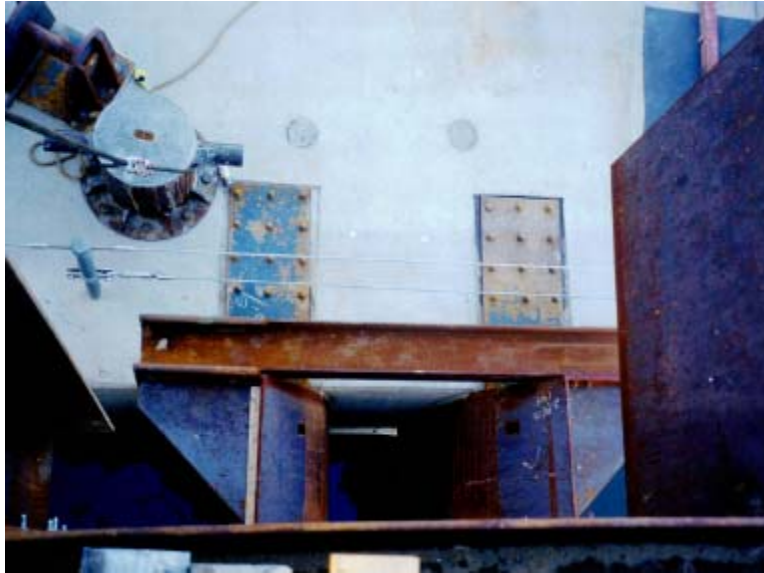
Figure A-38. Plan view of the horn-guide at Braddock Dam as the dam segment is ballasted to grade.
