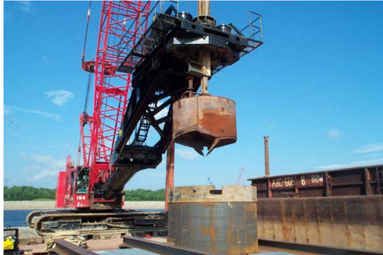
Figure A-117. Soil clean out with auger bucket.
