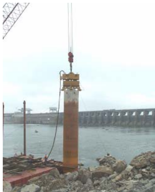
Figure A-116. Driving temporary casing.
