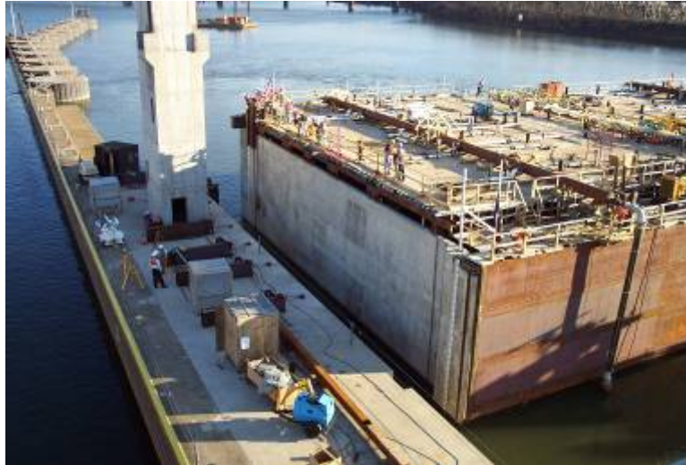
Figure A-36. Positioning Braddock Dam with guide attached to existing lock wall.
