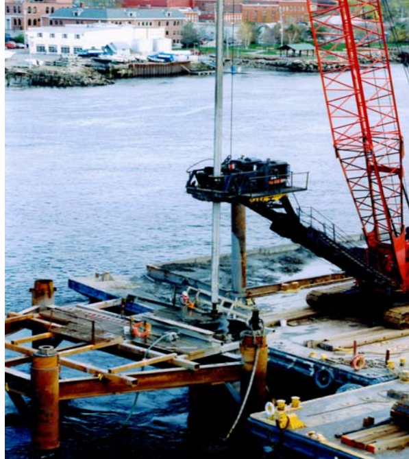
Figure A-39. Typical rotary drill rig Bath-Woolwich bridge.
