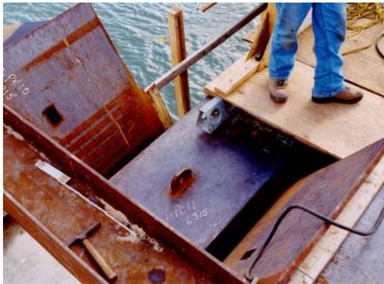
Figure A-3. Looking down on guide-arm as it enters horn-guide during landing of first dam segment at Braddock Dam.
