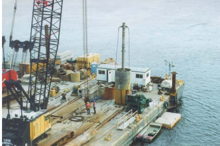
Figure A-41. Rotary barrel working over water.
