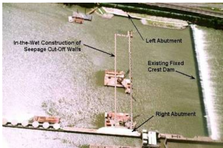
Figure A-77. Alignment of seepage cut-off walls.
