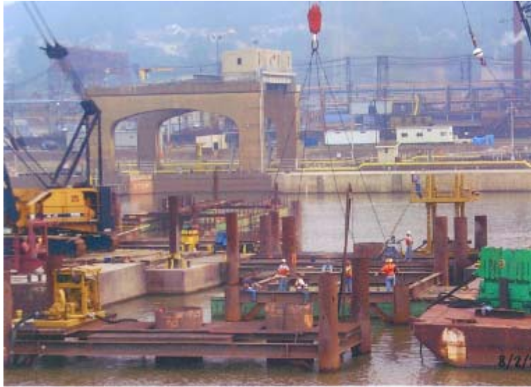
Figure A-87. Positioning drilled shaft templates.
