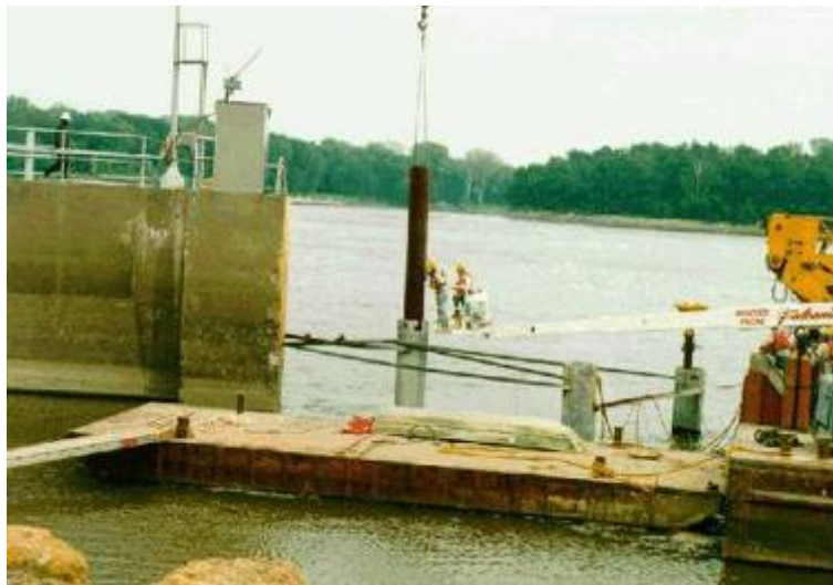
Figure A-104. Installation of a guide pile.
