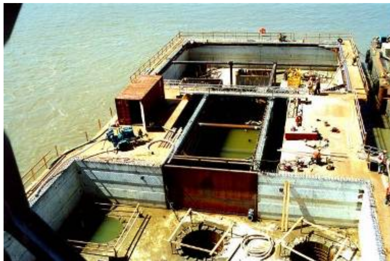
Figure A-10. Dewatered cofferdam and tops of drilled shafts at New Carquinez Bridge.
