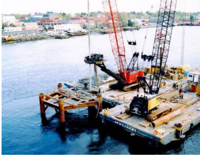
Figure A-33. Bottom founded template used to install drilled shaft casings at the Bath-Woolwich Bridge.
