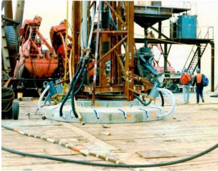
Figure A-19. Base of the guide tower leg before inflation of grout bags, Confederation Bridge.
