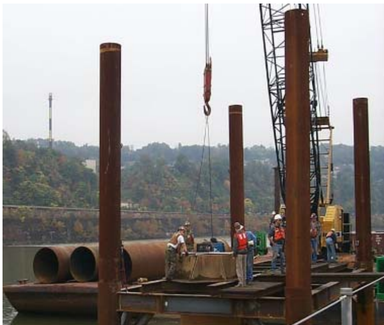
Figure A-88. Installation of template “guide tube.”
