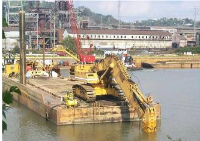
Figure A-76. Hydraulic backhoe dredging dam footprint.
