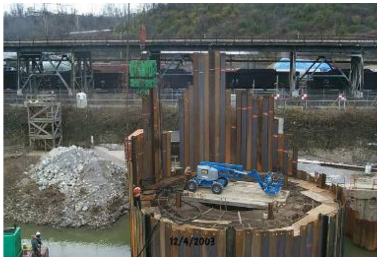
Figure A-101. Driving sheet pile cell for left closure weir.
