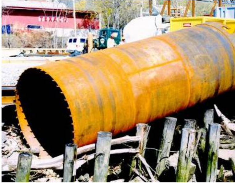
Figure A-42. Barrel with 72-inch diameter and cutters welded to bottom of casing to seat it into top of weak rock—Bath-Woolwich Bridge.
