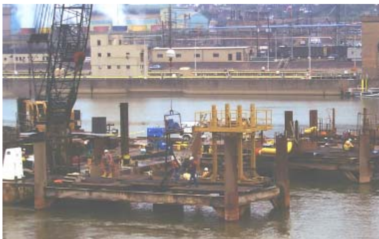
Figure A-92. Preparations for drilled shaft concrete placement.
