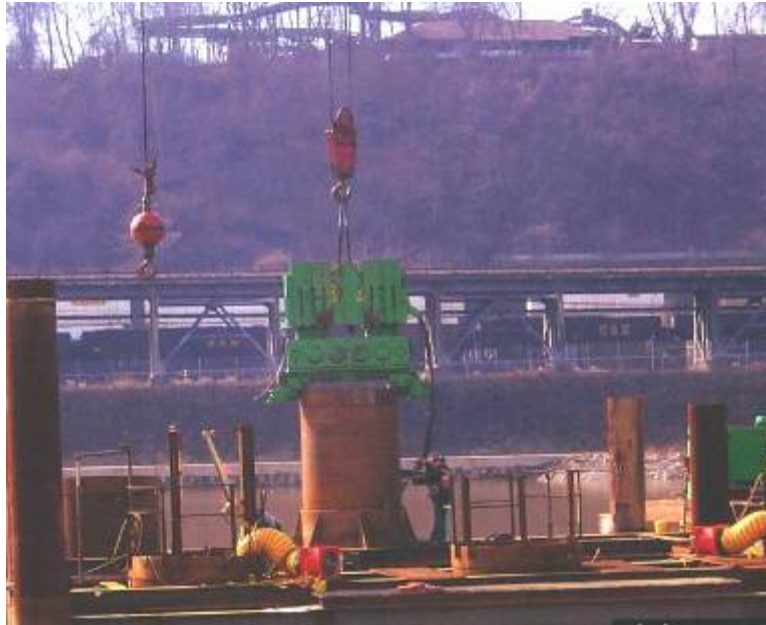
Figure A-89. Vibratory driving drilled shaft casing.
