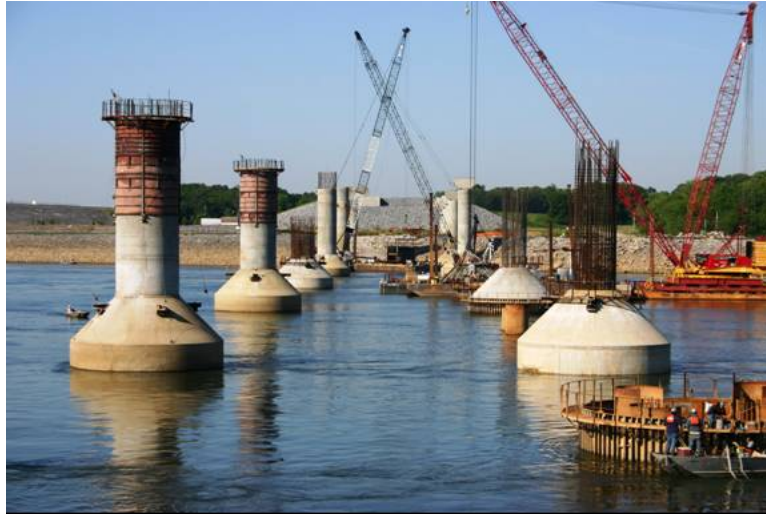
Figure A-130. Bridge piers.
