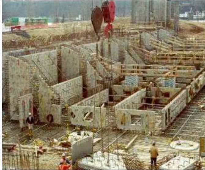
Figure A-5. Casting yard for Braddock Dam segments. See cylindrical block-outs in center.
