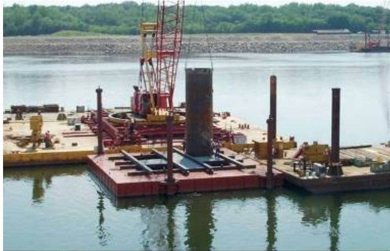
Figure A-115. Floating template.
