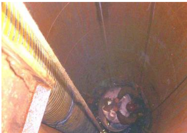
Figure A-95. Installation of shear pin inside dewatered casing.
